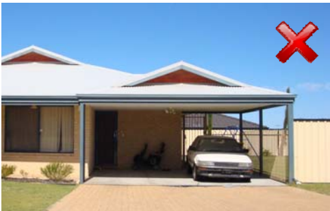
Incorrect: Brick walls with metal posts
