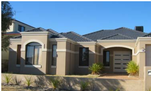
Two coloured feature walls with arched portico
