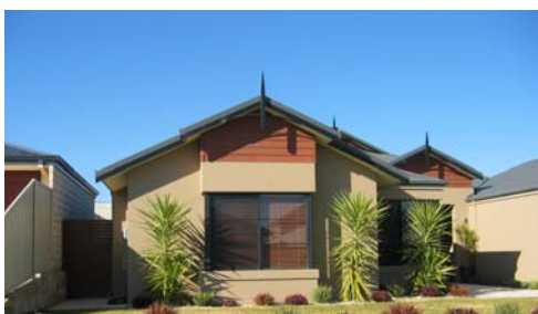
Gable with feature timber panelling
