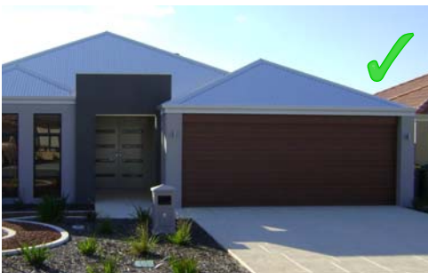
Correct: Rendered walls with rendered posts
