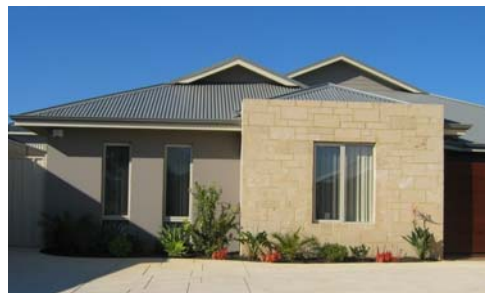
Contrasting wall materials
