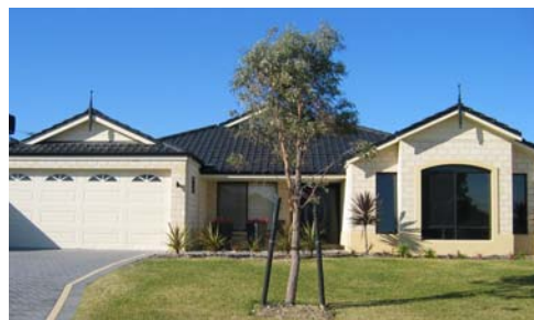
Gables facing the street
